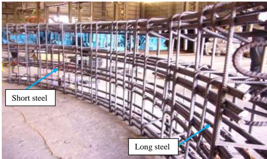
Figure 4. A fully assembled reinforcement steel cage for A1 panel.
