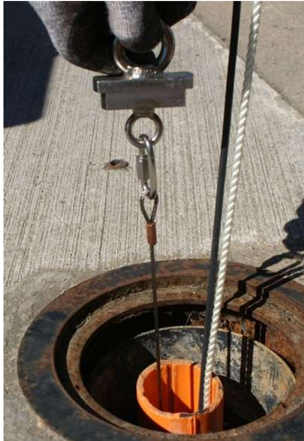
Figure 15: String lowered into hole with only top hanger, wire rope, support rope and cable visible
