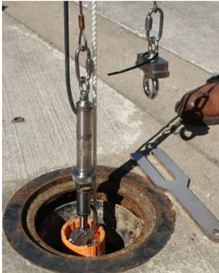
Figure 14: IPI string with top fly lead assembly fitted, being lowered into the casing
