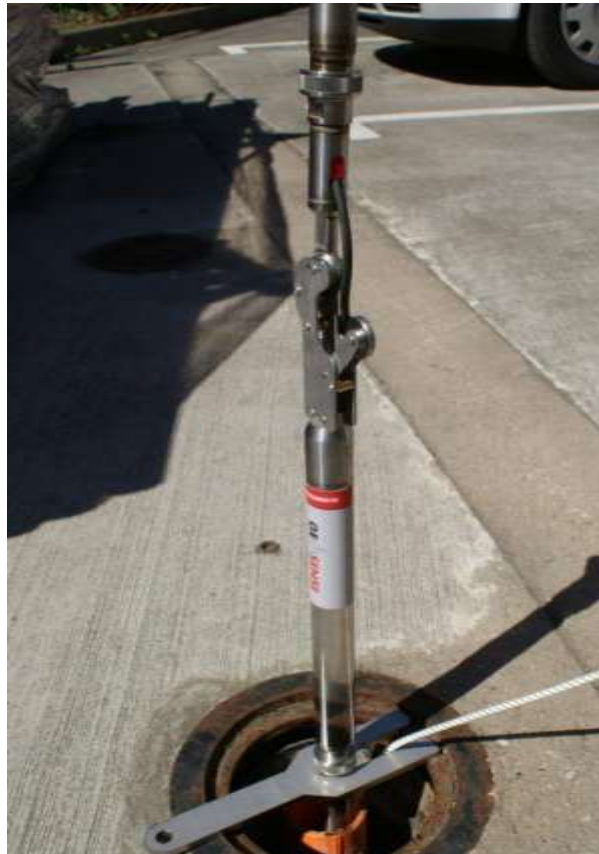
Figure 12: Sensors being added and locked off each time with the installation fork. The weight of the string when being lowered is held by the support rope. The sensor entering the hole can be aligned and held steady with a hand.
